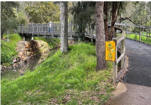
Figure 41: Safe Walkway Adjacent and Over Waterway
