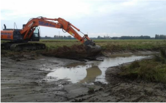
Figure 44: Waterfront Gradient Reduction Works
