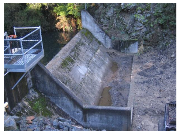
Figure 20: Low Head Dam / Weir
