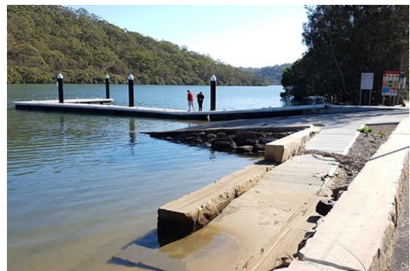
Figure 45: Jetty Constructed for Water Access
