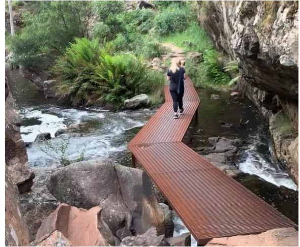
Figure 42: Walkway Over Waterway
