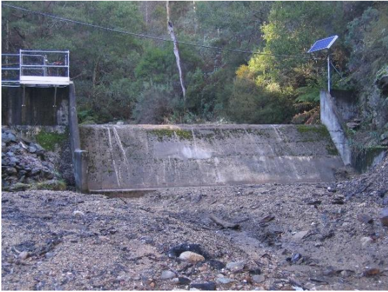
Figure 21: Low Head Dam / Weir
